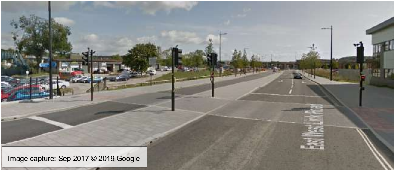
Figure 7-9 - Lincoln East West Link Road Toucan Crossing
