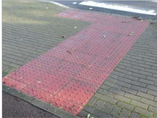
Figure 7-6 - Tactile Paving at a Controlled Crossing (Source: CIHT Designing for Walking, 2015)
